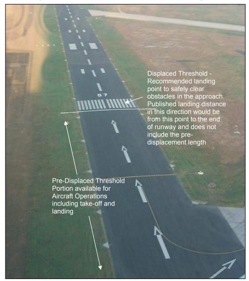
Figure 5-4 Sample Displaced Threshold Configuration<sup>5</sup>
